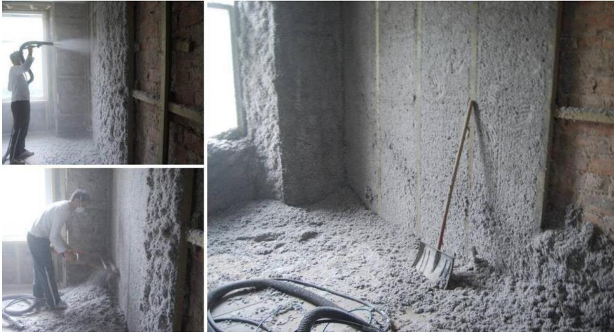
Figure 53 Cellulose fibre insulation is sprayed against the wall surface, lined with timber battens to receive a plasterboard finish.
