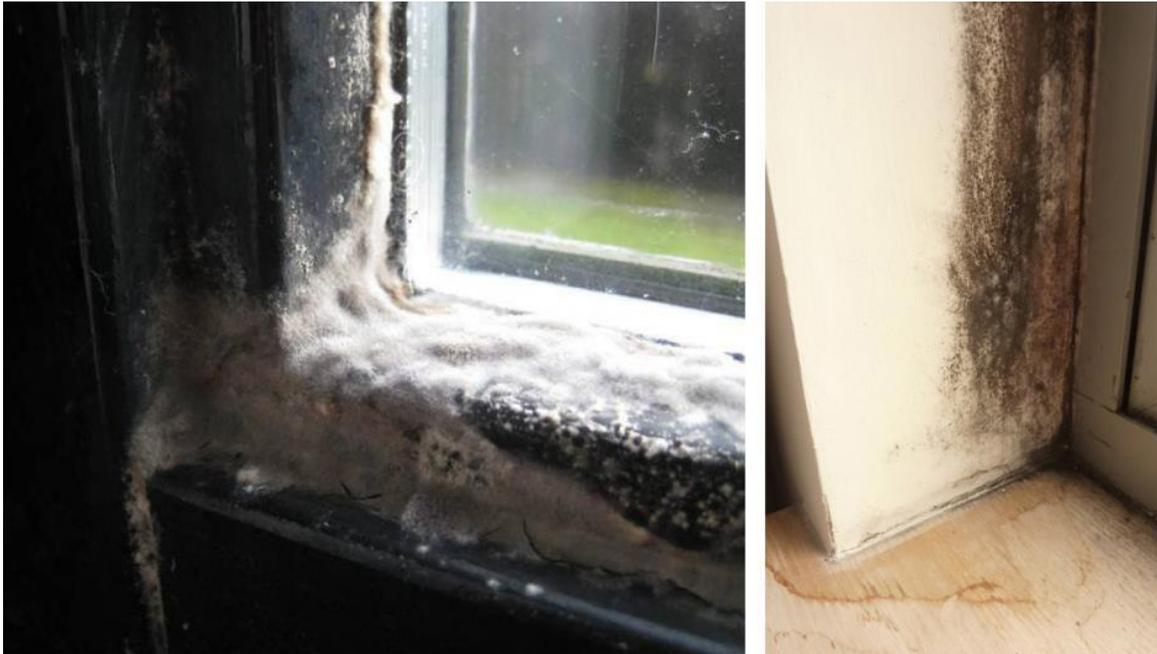
Figure 41 Severe mould growth on the non-hygroscopic surfaces of a coated window frame (left) and a plasterboarded window reveal (right).
