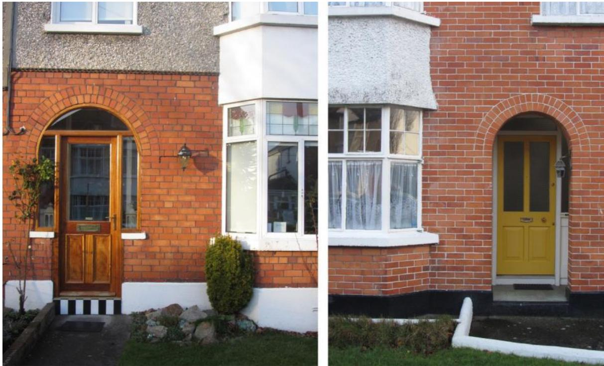
Figure 30 Two terraced houses either side of Skreen Road, Dublin, both built between 1936 and 1937: Despite using the same aesthetics and materials, the left building is a solid masonry wall, whereas the right building has a cavity wall.
